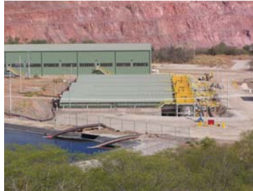
PV uses gravity flow of PLS
