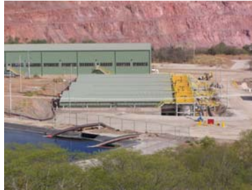
PV uses gravity flow of PLS
